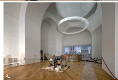
1. Musée National de la Marine, Paris. Renovation worksite. Palais de Chaillot. Davioud Gallery. 11/01/2023; h2o architectes and Snøhetta. © Patrick Tourneboeuf/OPPIC/Tendance Floue 2. Musée National de la Marine, Paris. Renovation worksite. Palais de Chaillot. Main Pavilion; Davioud Gallery. 11/01/2023; h2o architectes and Snøhetta. © Patrick Tourneboeuf/OPPIC/Tendance Floue.
